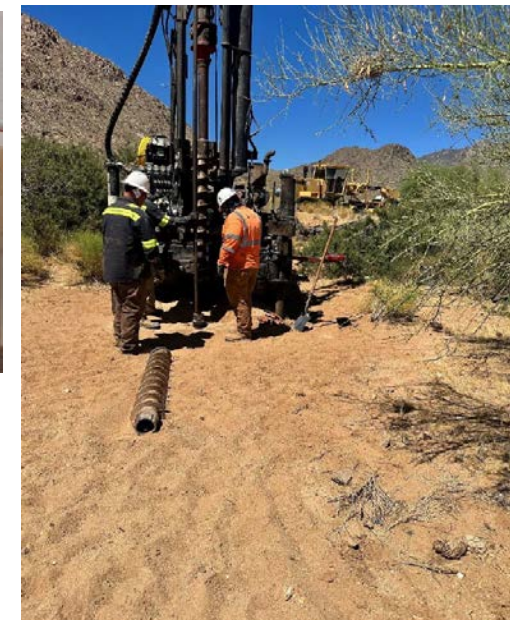
Surface Geotechnical Investigation – Cascade Drilling
